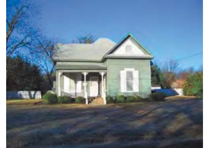
Appropriate Colors for a Folk Victorian House (simple paint scheme with a single trim color used)
