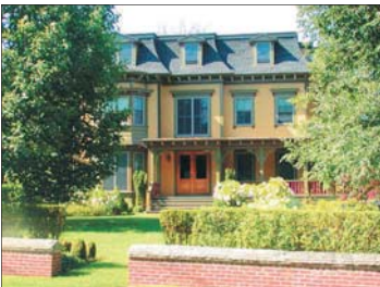
Second Empire style home with a lively and contrasting paint scheme; a different color is for chosen for different levels of trim to create a vibrant effect, which was popular when this home was built.
